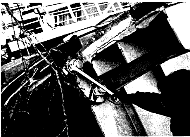
Fig. 38. Failed tension link on a collapsed rail span.
